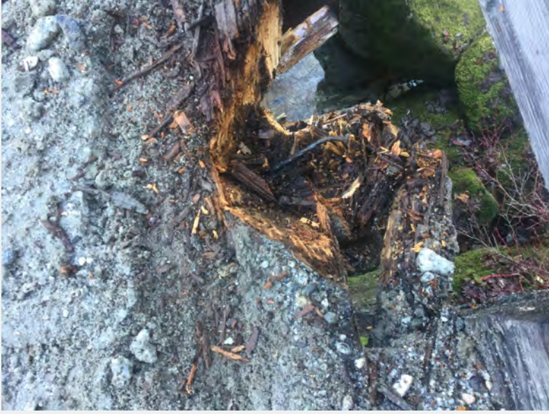
Timber deck condition along deck edge
