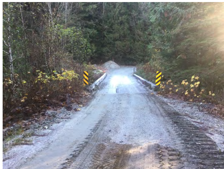
Approach from Right Bank when facing downstream
