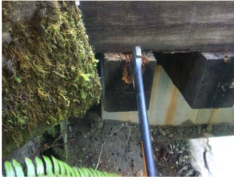
Typical cross tie condition at ends
