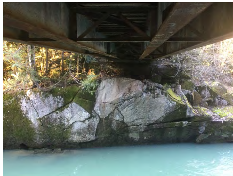
Right Bank Abutment when facing downstream
