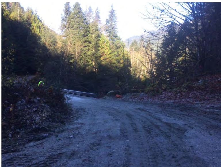
Approach from Left Bank when facing downstream
