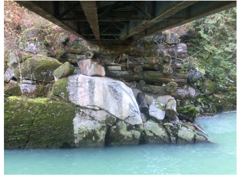
Left Bank Abutment when facing downstream
