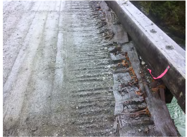
Recent track equipment passing over bridge
